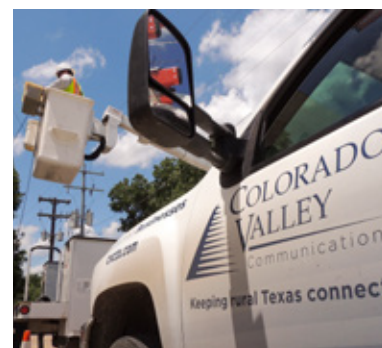
Above: CVCTX installer Chris Janacek connects an aerial service from his bucket truck.
